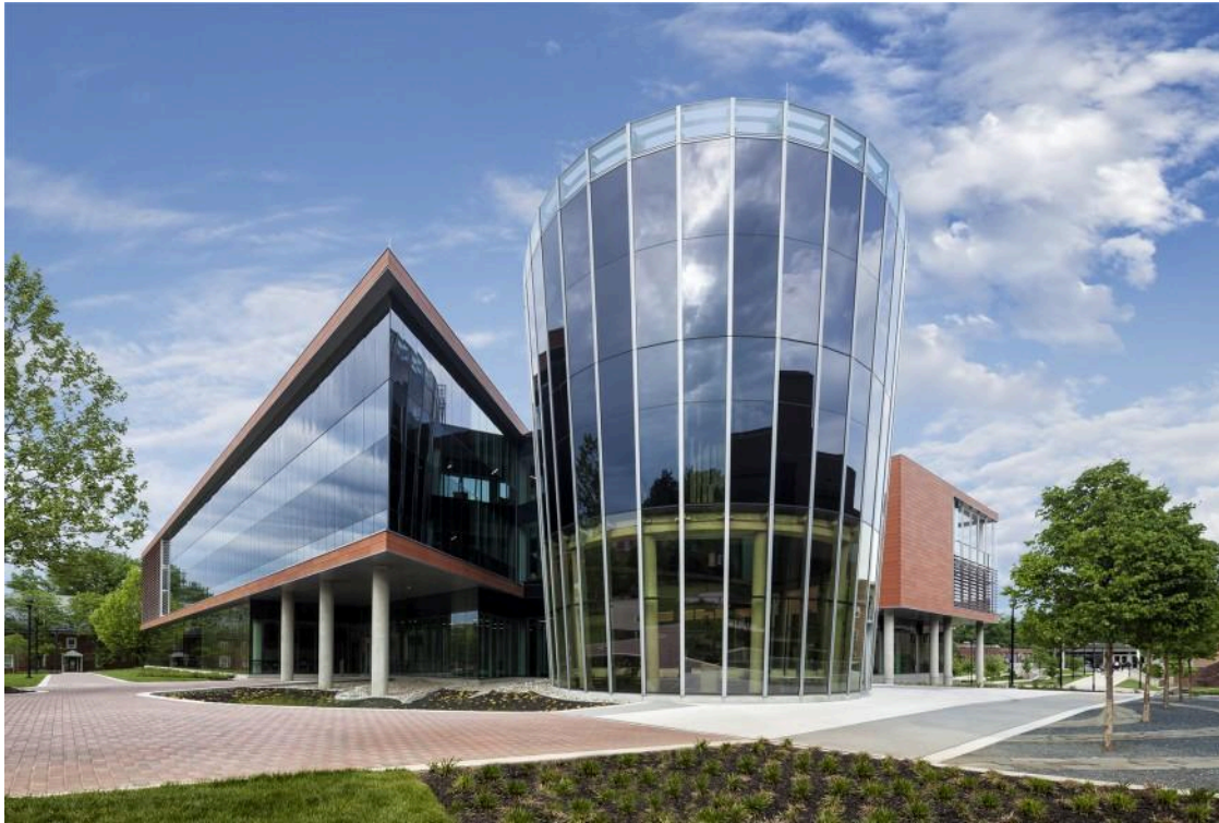
Center for Natural Sciences, Mathematics, and Nursing at Bowie State University, Md. (Photo courtesy of SageGlass)
