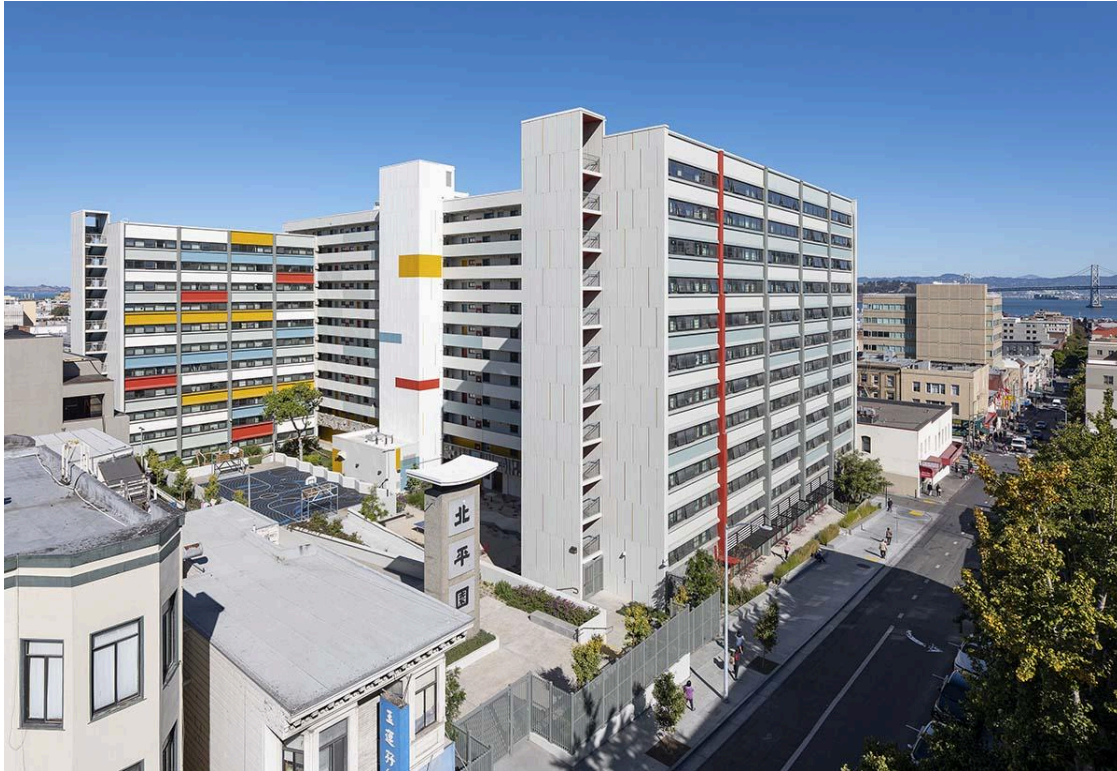
Ping Yuen North in San Francisco, Calif. (Photo courtesy of Gelfand Partners Architects)
