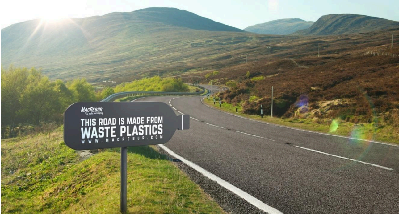
Plastic-paved roadway (Photo Courtesy of MacRebur)
