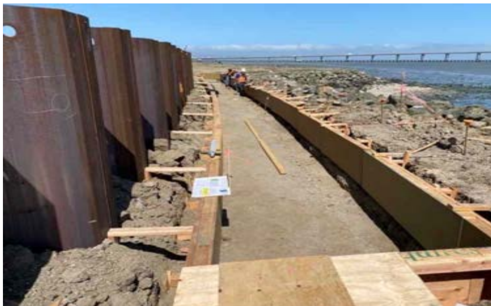
Construction of a seawall in Foster City, Calif.
