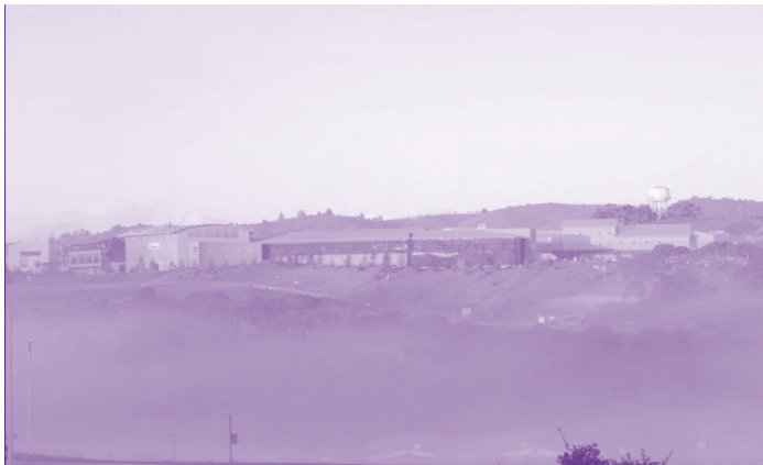
San Mateo County's new energy-efficient Youth Services Center. Photo courtesy of San Mateo County.
