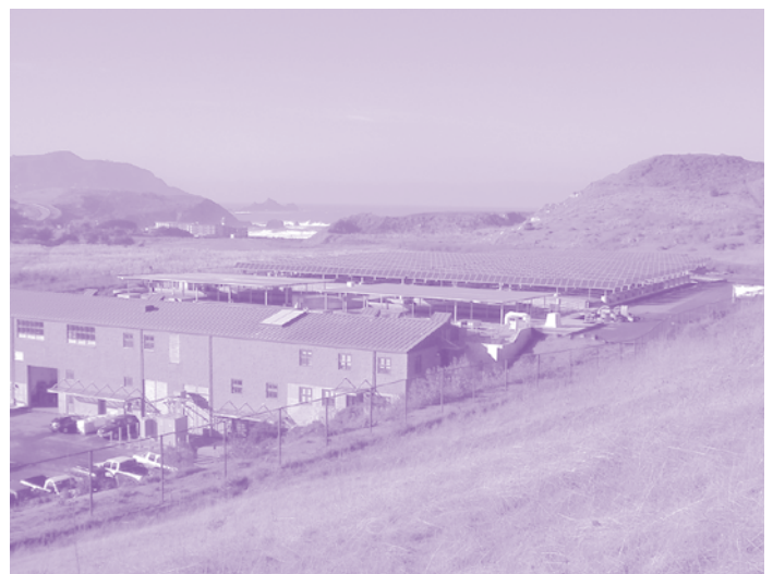
The City of Pacifica's Calera Creek Water Recycling Plant, a SSMC 2000 Award Winner. Photo Courtesy of the City of Pacifica.
